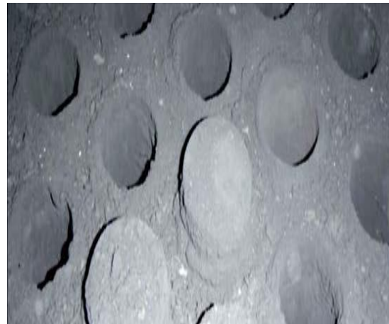
Eroded tube terminations adjacent to plugged tubes
