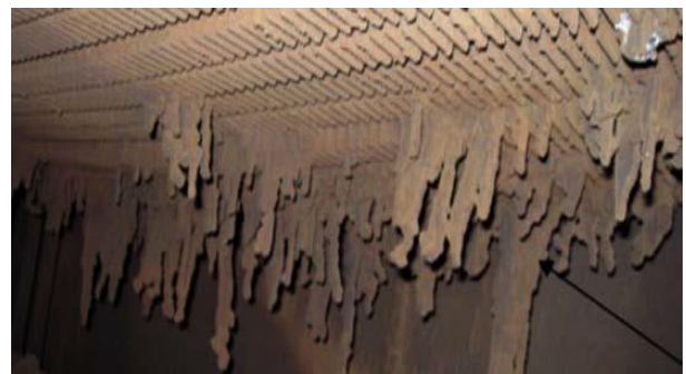
Exhaust gas boiler soot fire: melted uncooled fin tube elements
