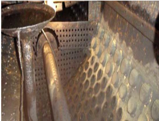
Excessive local plugging in steam drum
